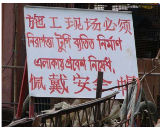
Fig-19: Notice in the bridge site
