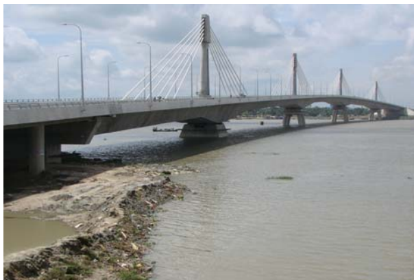
Fig-22: Completed Third Karnaphuli Bridge
