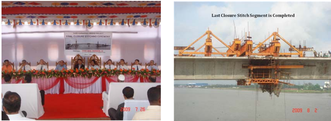
Fig-21: Final closure stitching of Third Karnaphuli Bridge
