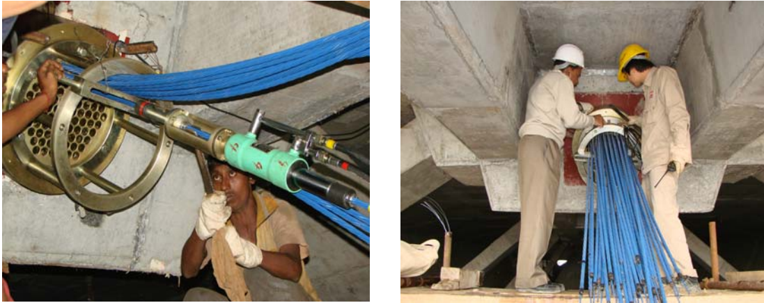
Fig-9: The deck anchorage of stay cable of Third Karnaphuli Bridge
