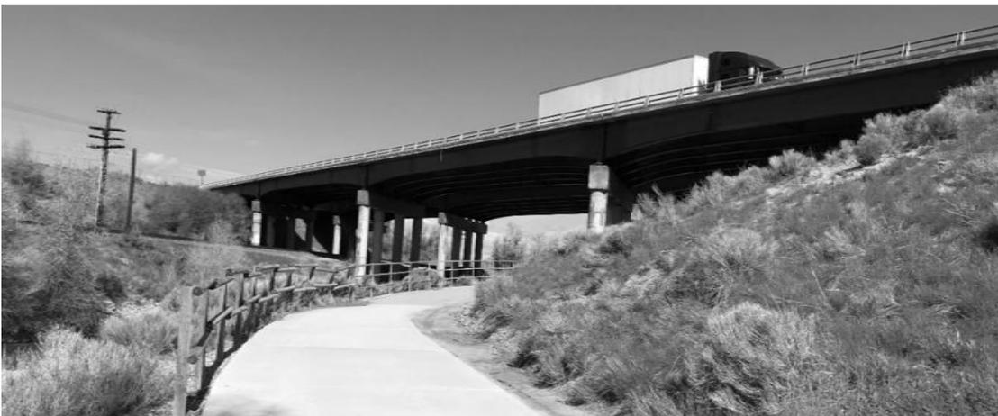
Figure 1. Skewed four-span concrete slab on steel girders highway bridge along I-80 in Evanston, Wyoming.
