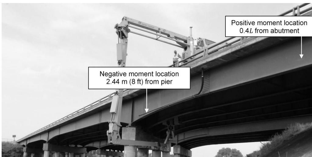
Figure 3. Instrumentation of the steel girders at the positive and negative moment locations.
