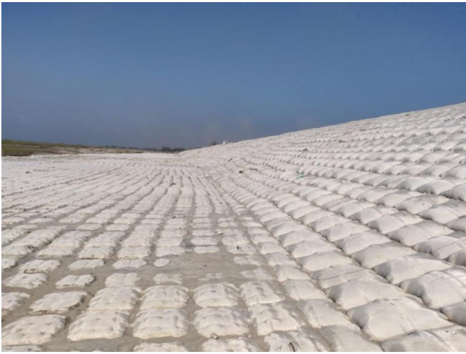
Figure 4. Articulating block concrete mattress after installation at site.
