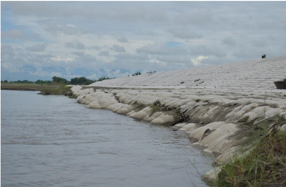
Figure 6. Articulation of the concrete block mattress recorded at site.
