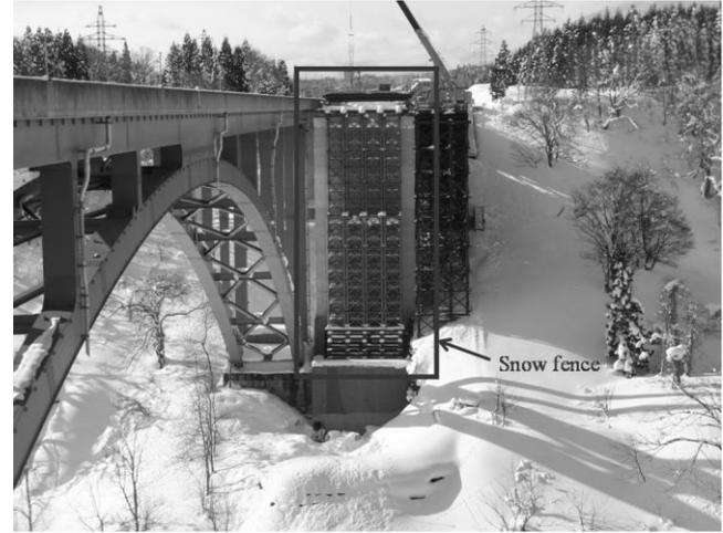
Figure 9. The distribution of the maximum axial strain generated. Figure 10. Installed snow fence.
