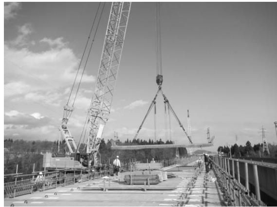
Figure 19. Floor slab erection.
