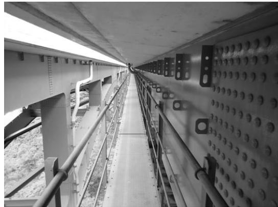
Figure 21. Inspection road of arch crown.
