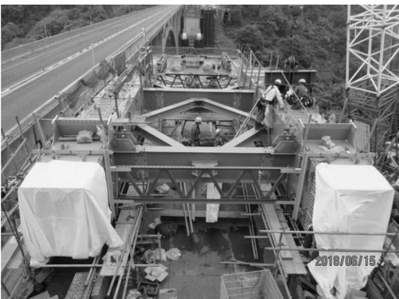
Figure 16. Suspended by the two erection cable.
