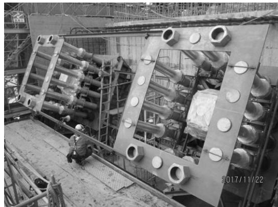
Figure 23. Arch-base anchor bolts with hot-dip galvanized.
