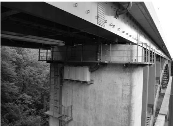
Figure 22. The oil/water separator on the pier.
