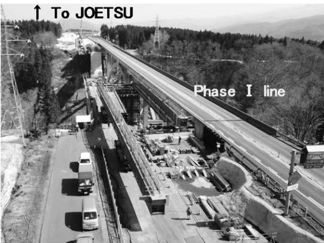
Figure 11. Transportation by multi-axle trolley.
