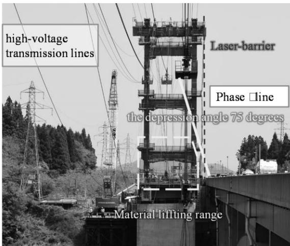
Figure 14. Setting of the material lifting range.
