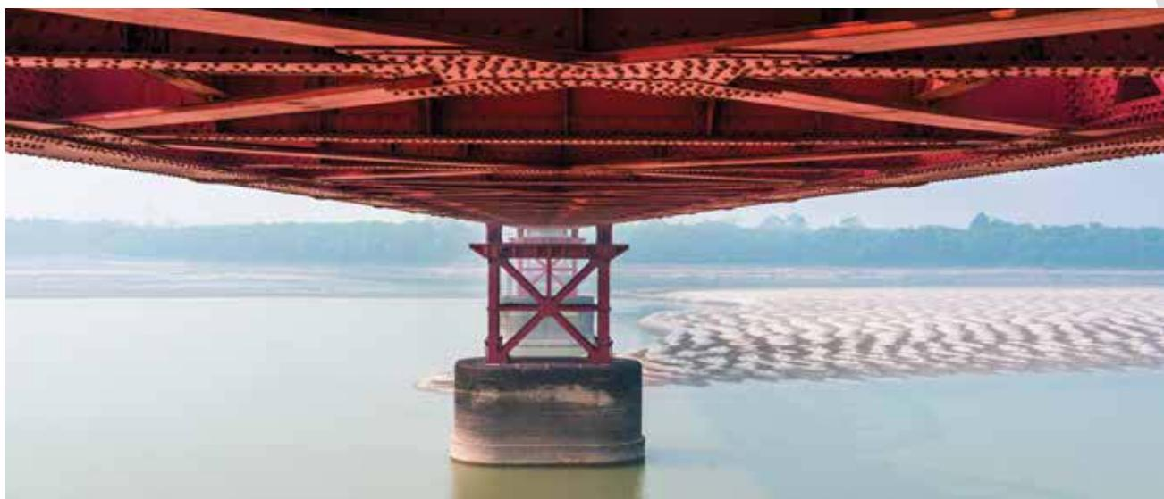
Photo 3. Bherama end of the Hardinge Bridge today showing siltation but no erosion. Images by: A.F.M.S. Amin
