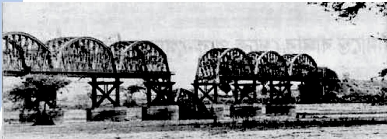
Photo 4. The photograph of Hardinge Bridge showing the fallen Span 12. Image from Internet
