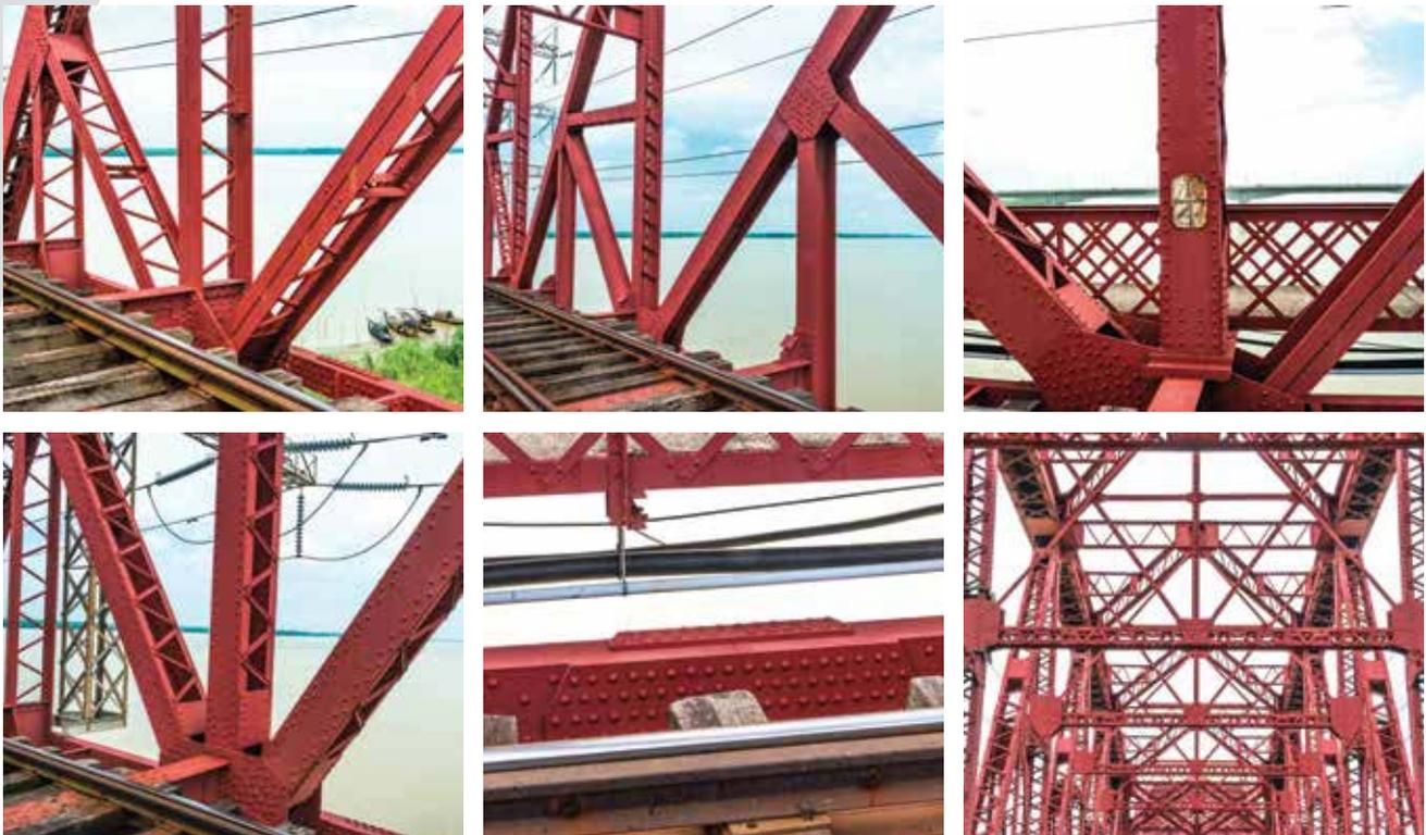
Photos 5-10. The photographs depict the repair work of Span 9 and Span 12 after 1971 war damage. Images by A.F.M.S. Amin.
