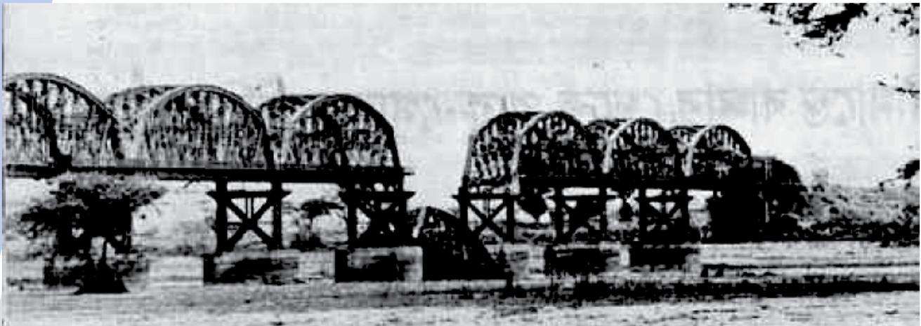
Photo 4. The photograph of Hardinge Bridge showing the fallen Span 12. Image from Internet
