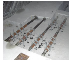
Figure 12. Installation of the anti-jumping steel hoops
