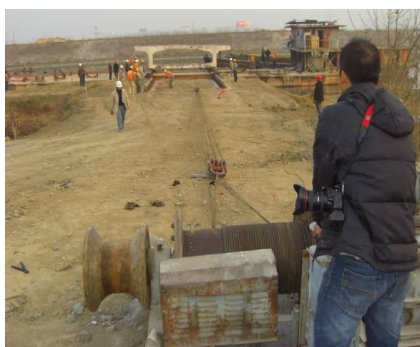
Figure 19. Dragging the section of box girder by winch hauling system
