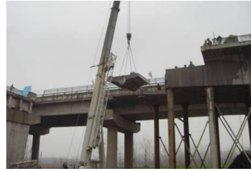
Figure 22. Sections of the side spans hanged in blocks
