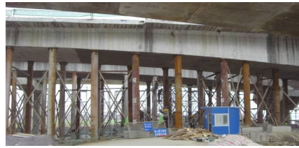
Figure 10. After the steel pipe support prepressing
