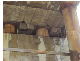
Figure 14. Steel drums between the main pier and the beam
