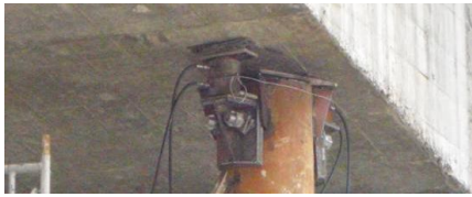
Figure 9. Scene of the steel pipe support prepressing
