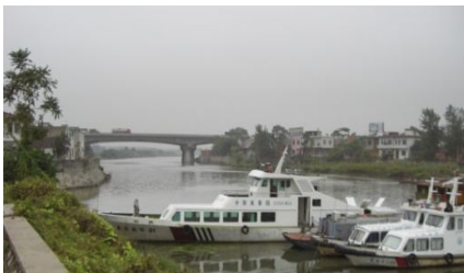
Figure 1. The old Nanfeihe Bridge
