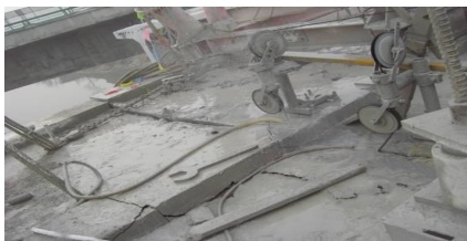
Figure 4. Concrete being cut by chain-cutter
