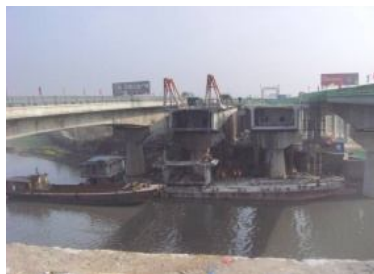
Figure 17. Drop the mid-span of box girder
