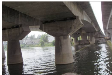
Figure 2. The old Nanfeihe Bridge
