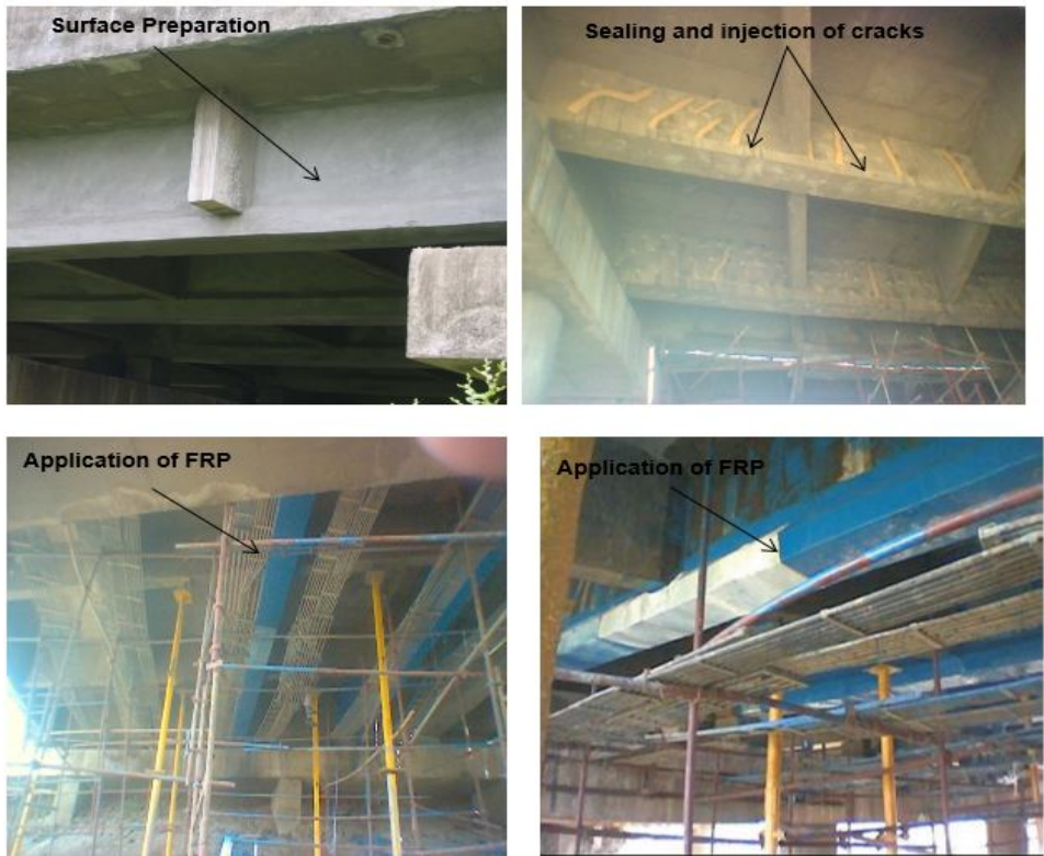
Figure 3. Application of FRP composite on Chaltan Bridge
