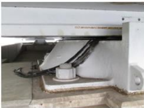
Picture 3. Re-Damage of Movable Bearing
