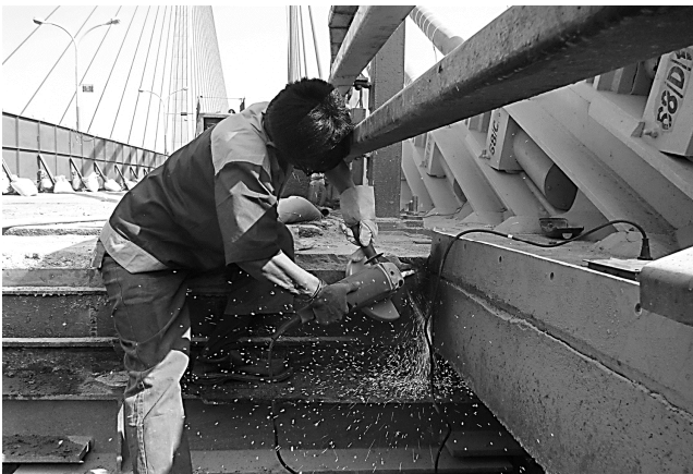
Figure 11. Surface preparation of the steel side of Modular joint
