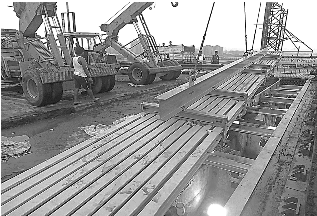
Figure 15. Positioning of Lamella beam assembly
