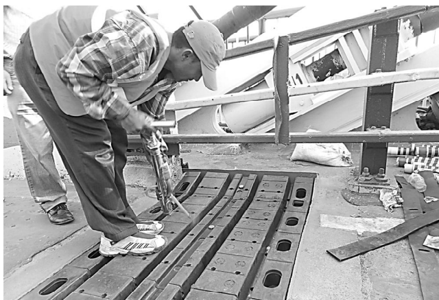
Figure 9. Fixing of new slabs in position
