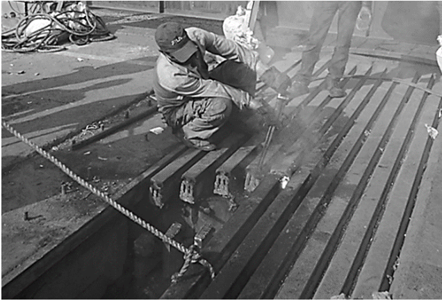
Figure 10. Removal of existing joint
