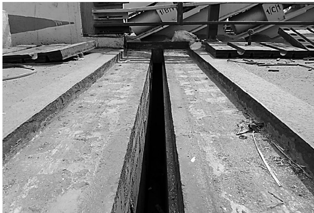
Figure 8. Prepared surface for placing new slabs
