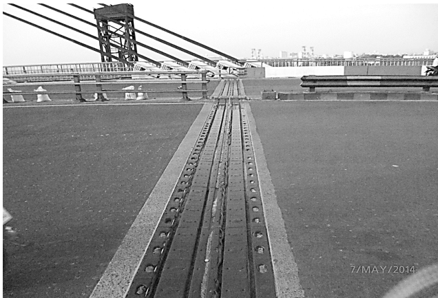
Figure 3. Existing Slab Seal (matt) joint
