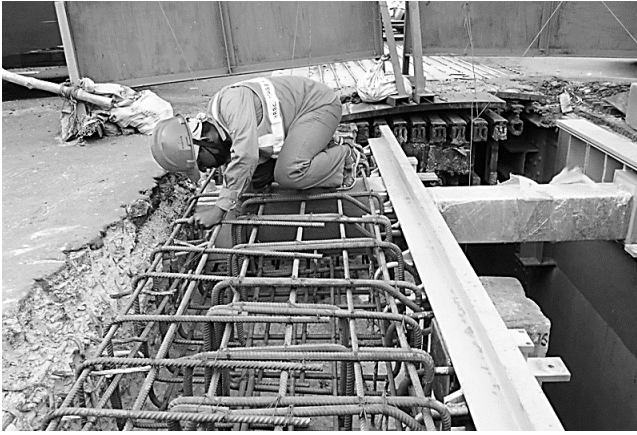
Figure 12. Prepared concrete recess of new Modular joint
