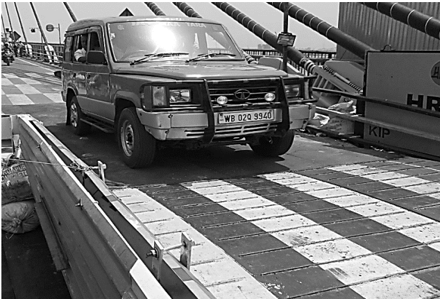
Figure 6. Traffic plying over Bridging Plate
