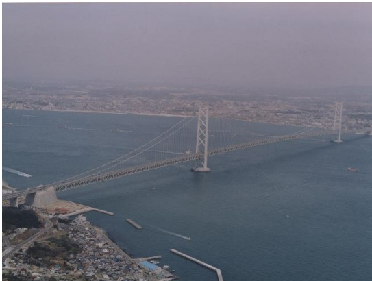
Figure 1. Akashi Kaikyo Bridge
