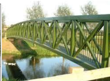
Tubular Truss Bridge, UK
