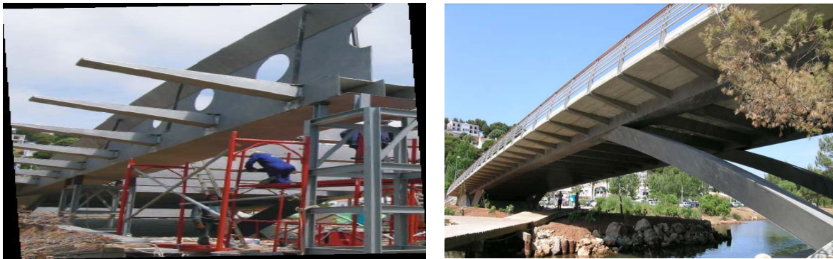
Figure 2. Cala Galdana Road Bridge, Menorca, Spain 2005 (Baddoo, and Kosmac 2013)
