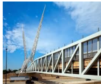
Tubular Bridge Oklahoma City
