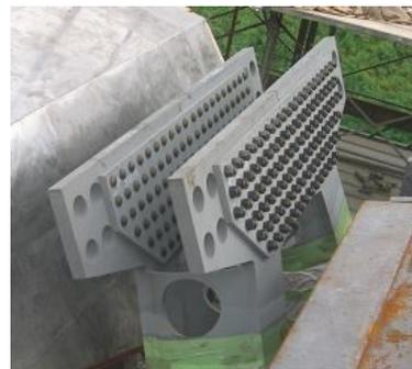
Figure 7. Double friction gusset joint system
