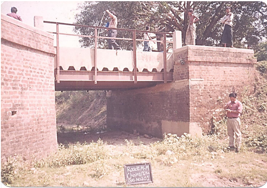
Figure 1. Steel through plate Bridge at Modhupur-Mymensing Highway
