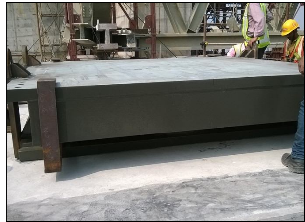
Figure 18. Placement of bearing over anchor plate
