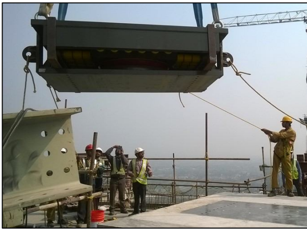
Figure 17. Lifting of bearing of approx. wt. 15T
