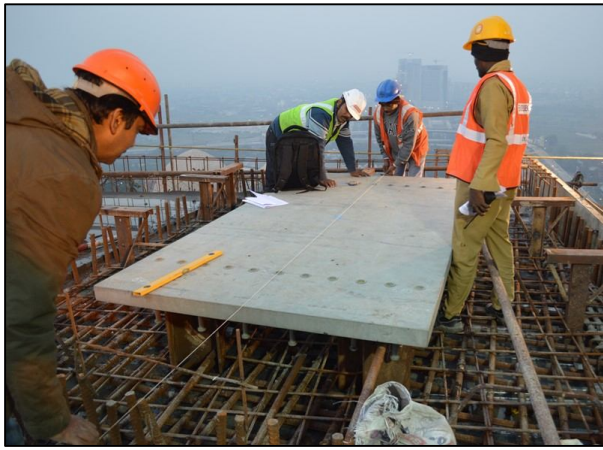
Figure 15. Placement of anchor plate
