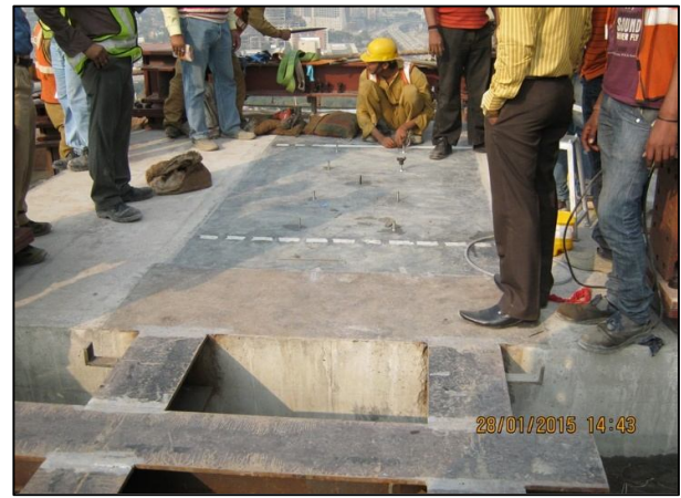
Figure 16. Pressure grouting below anchor plate
