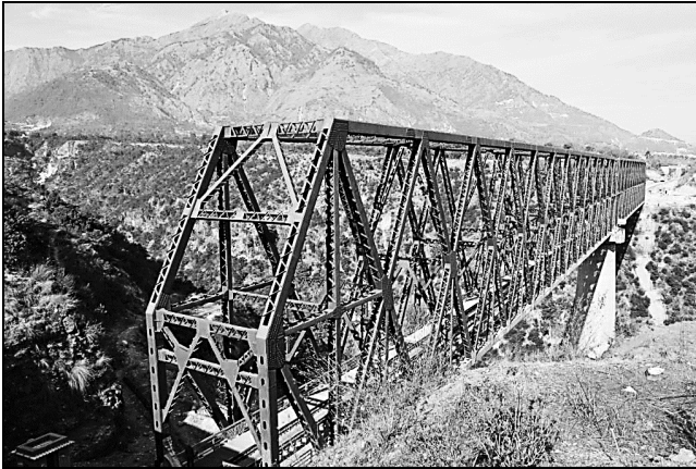
Figure 10. Bridge No. 20 at a height of 85 metres, Asia's tallest steel railway bridge
