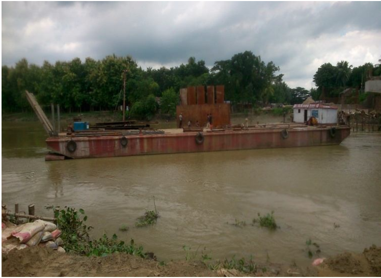
Figure 6. Placing of prefabricated steel coffer dam
