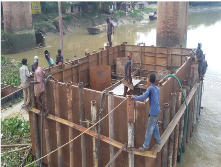
Figure 7. Watering, De-watering & Anchoring of prefabricated steel coffer dam
