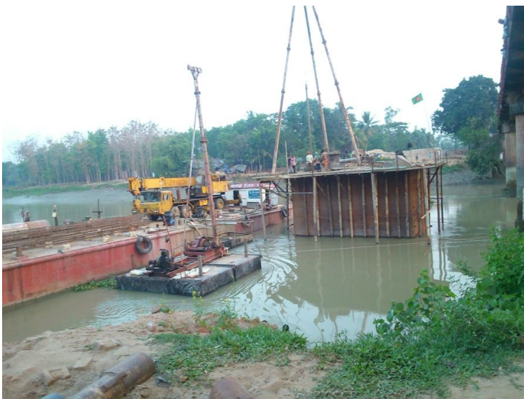
Figure 8. Construction of Pile over prefabricated steel coffer dam
