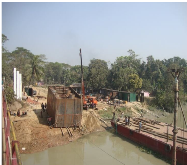
Figure 5. Photographs of prefabricated steel coffer dam
