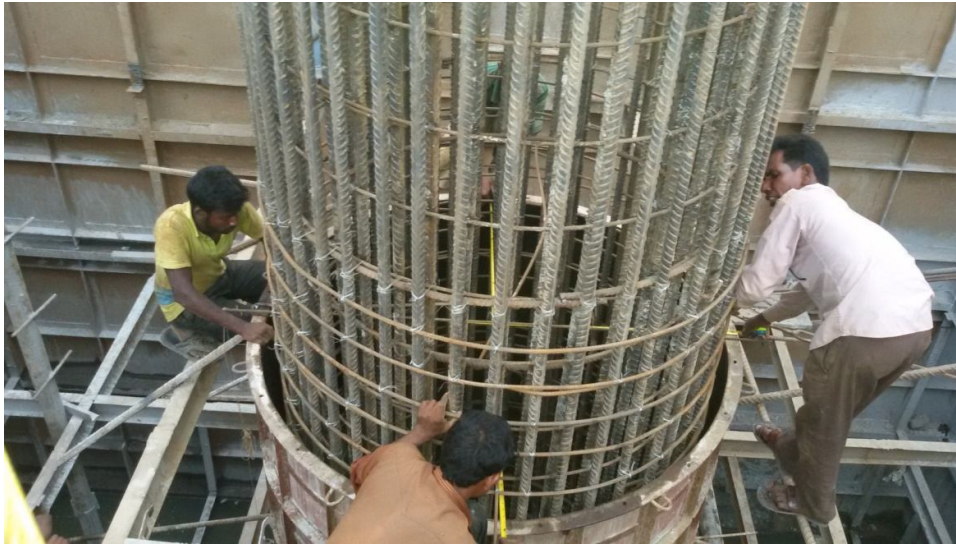
Figure 9. Construction of pier shaft inside prefabricated steel coffer dam
