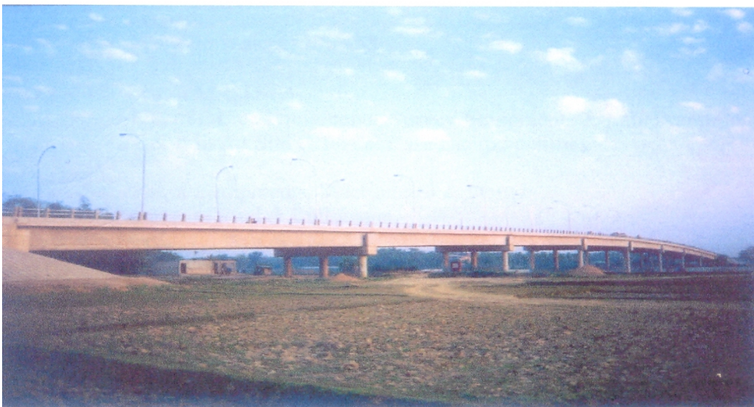
Fig. 1 Photograph of the completed Hazrat Shah Paran (r) Bridge
