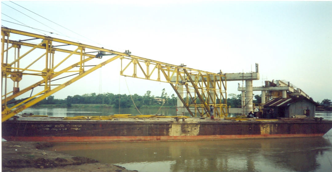
Fig. 5 Erection / dismantling system of truss modules
