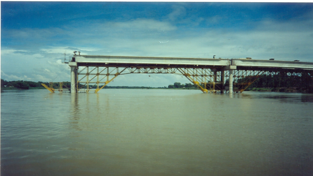
Fig. 4 Photograph shows the system of erected truss supports during monsoon season
