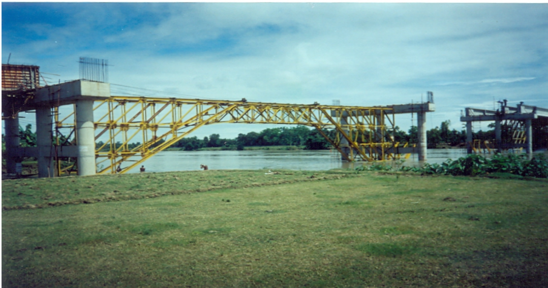
Fig. 3 Bridge girder construction by using triangular space truss support
