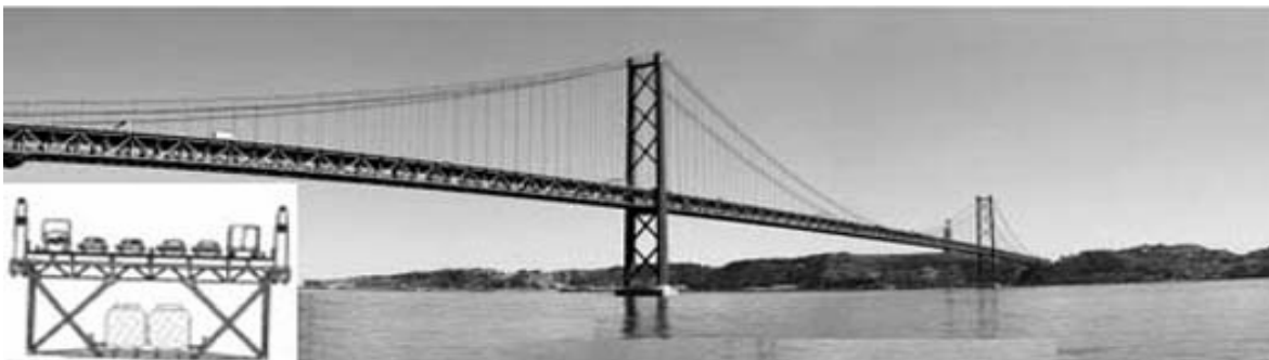
Figure 3: The Tagus River Bridge, Lisbon, Portugal
