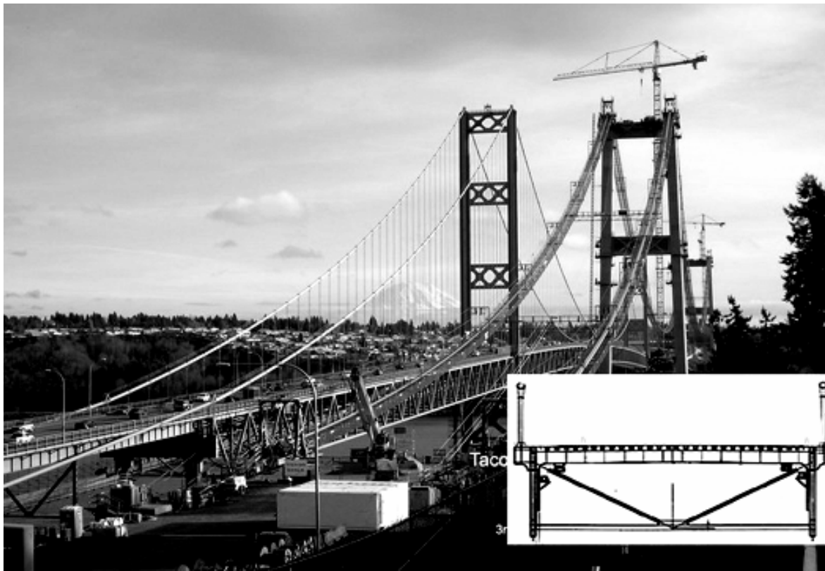
Figure 4: The Third Tacoma Narrows Bridge, Washington, USA
