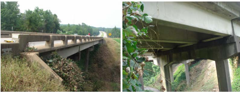
Figure 2. Overview of bridge on highway I-78
