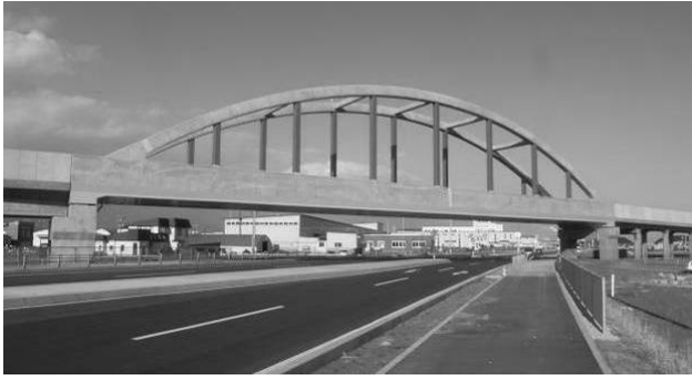
Figure 1. Steel-concrete hybrid PC Langer bridge
