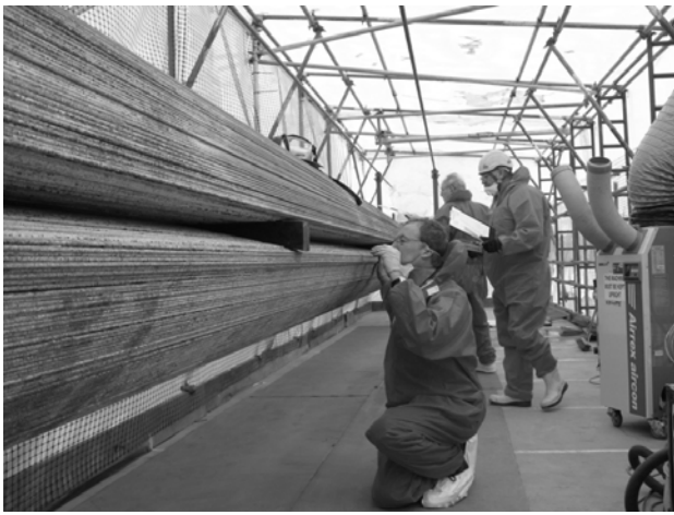
Figure 2: Inspecting the 3:00 o'clock wedge line
