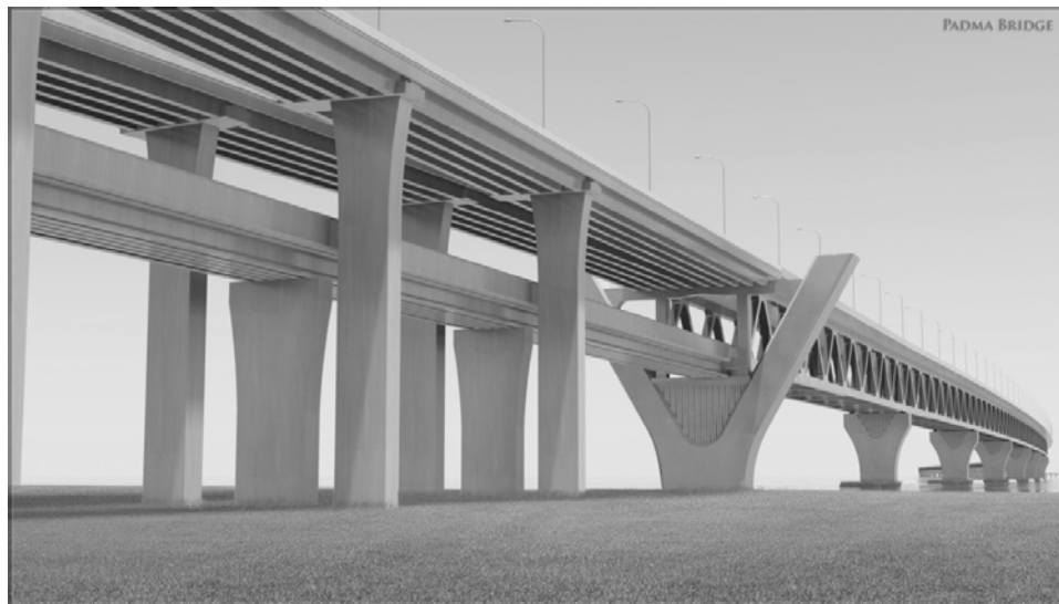
Figure 6. Transition Pier between Main Bridge and Approach Viaduct will be used as access and also as an emergency evacuation route.
