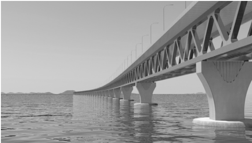
Figure 3. View of the preferred option: two-level steel truss bridge
