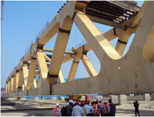
Figure 4. A Fabricated total span of the bridge.
