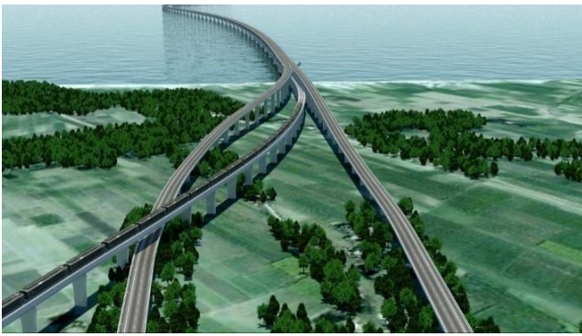
Figure 6. Arrangement viaduct at Mawa end.
