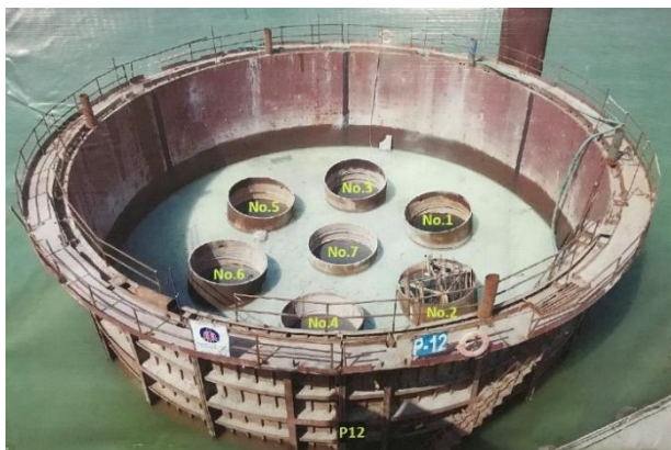
Figure 2. Arrangement of 6-pile cluster.
