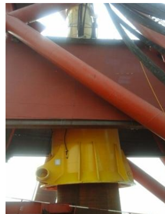
Figure 12. Driving of Piles at 1:6 slope.
