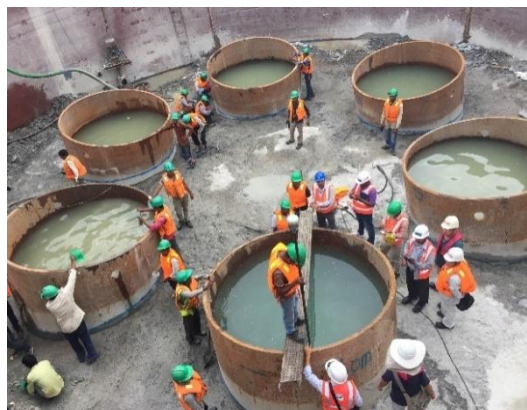
Figure 3. Arrangement of 7-pile cluster.
