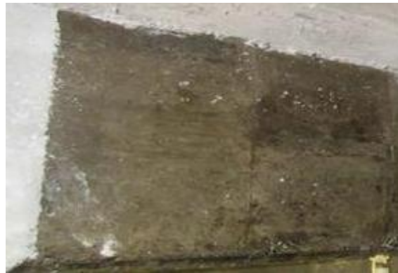
Figure 5. Adjustment of unevenness with putty.
