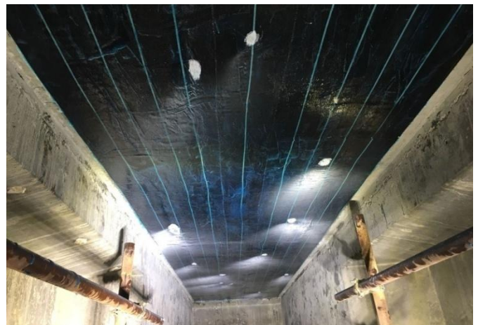
Figure 11. Bridge deck slab after applying CFRP.
