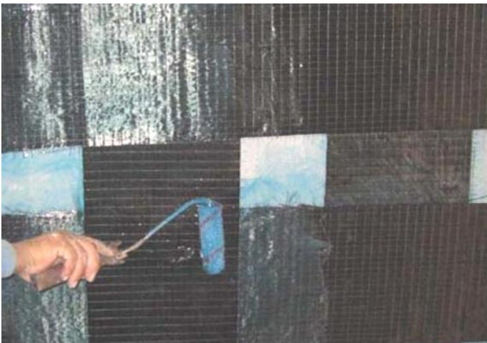
Figure 8. Squeezing of strip to entrapped air.
