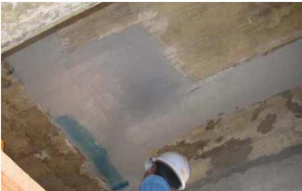
Figure 4. Adjustment of unevenness with putty.
