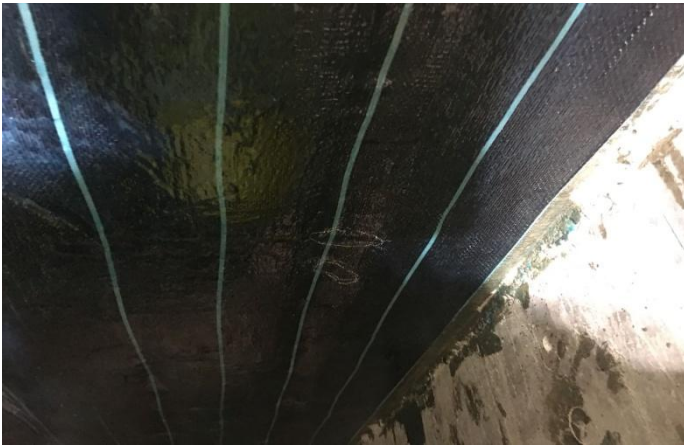
Figure 6. Putting longitudinal layer of CFS.
