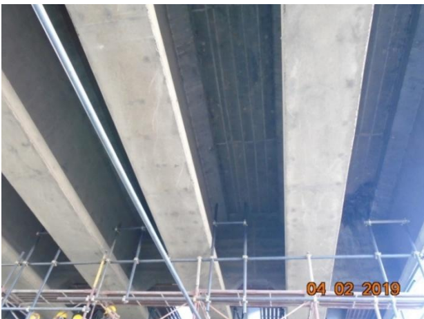
Figure 10. Bridge deck slab before applying CFRP.
