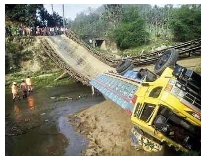
Figure 2. Bailey bridge collapse in Bandarban (The Independent, 2016)
