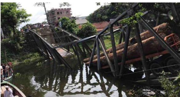
Figure 1. Bailey bridge collapse in Munshiganj (UNB, 2020).
