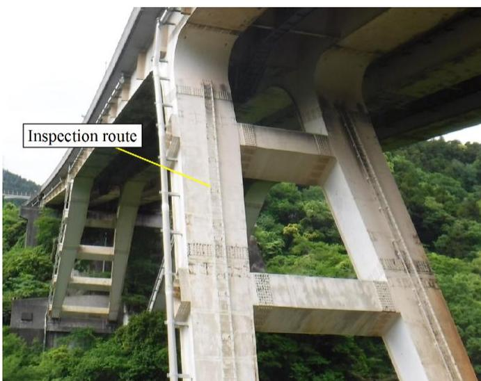
Figure 8. Status of inspection route before seismic reinforcement work.
