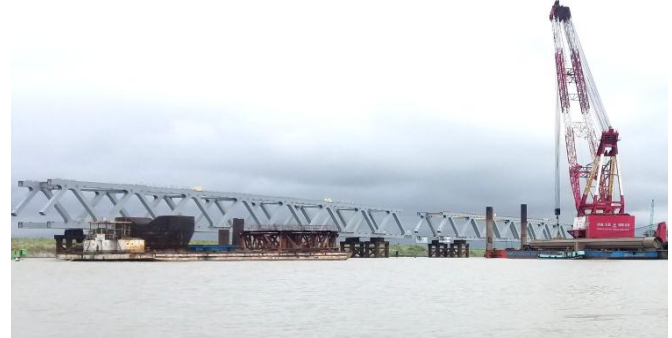
Figure 33. Two truss spans in 'storage' on piled supports.
