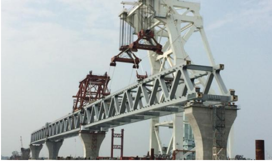
Figure 9. Erection of subsequent spans along module.
