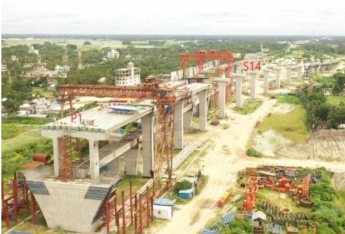
Figure 32. View of the Mawa viaducts.
