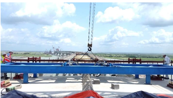
Figure 26. View of the erection front along Module 7.
