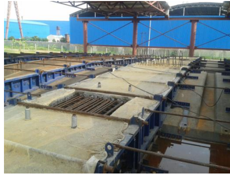
Figure 17. Curing of panels in casting bed.
