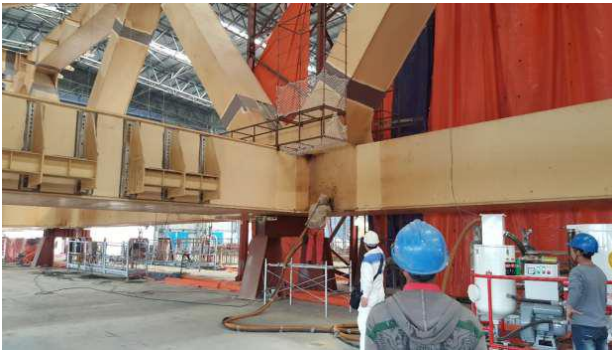
Figure 14. Truss in painting shop.
