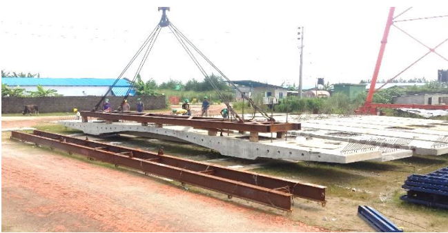
Figure 19. Lifting panels from casting bed.
