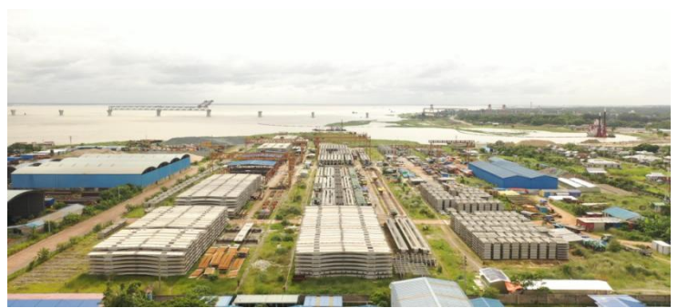
Figure 20. Mawa storage yard showing large storage requirements for road and railway panels.
