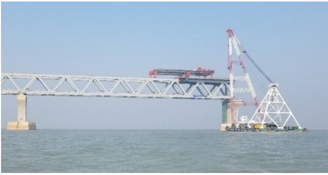
Figure 28. LG2 commencing along Module 3.
