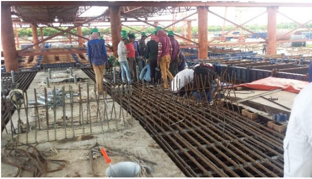
Figure 16. Prefabricated reinforcement cage in casting bed.
