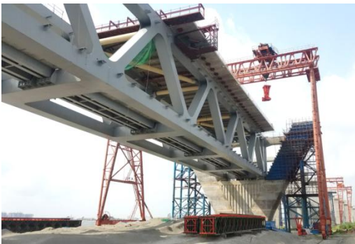
Figure 24. First deck panels erected by gantry.
