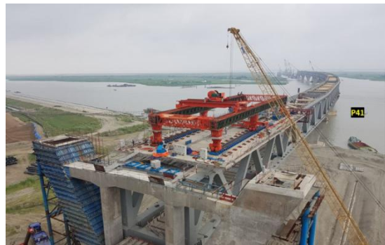
Figure 25. Erection of LG1 onto first set of panels.
