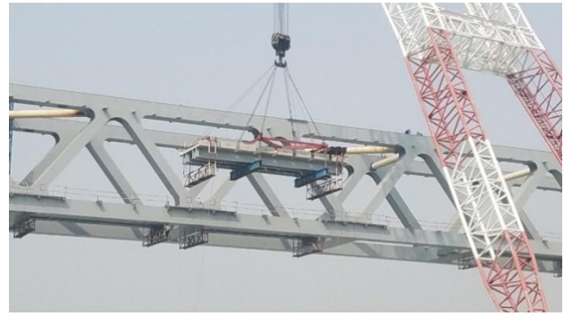
Figure 29. Erection of railway panel assemblies.
