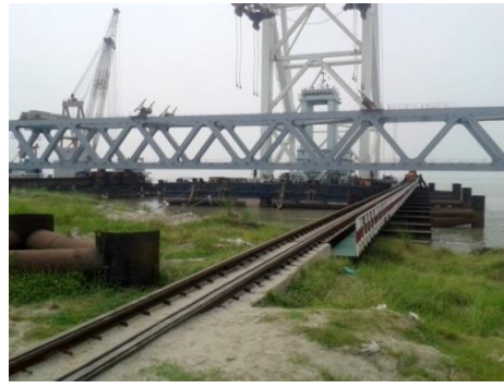
Figure 15. Loading out of truss onto floating crane Tian Yi.
