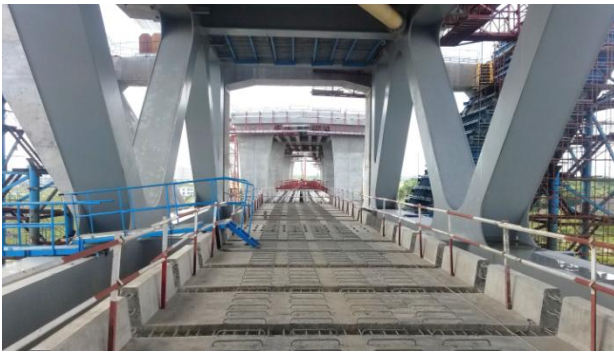
Figure 30. View along erected railway slab.
