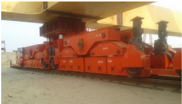
Figure 13. Special bogies for moving complete truss assemblies.
