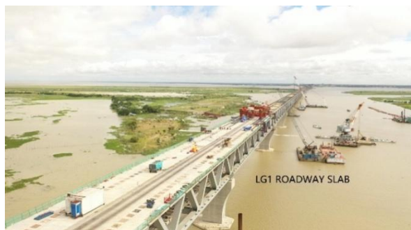
Figure 27. View of LG1 progressing along Module.
