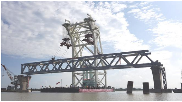
Figure 8. Erection of first spans of module.
