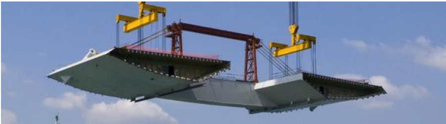
steel orthotropic deck
