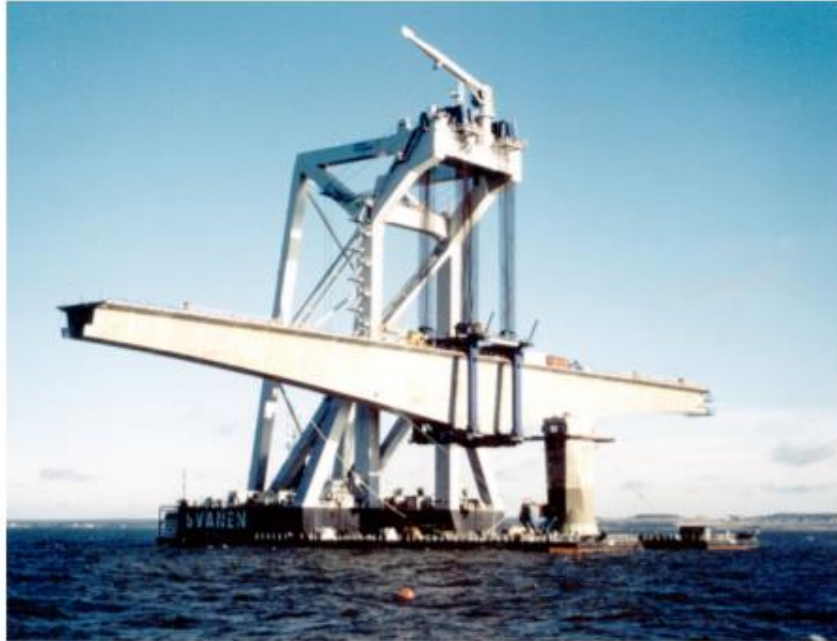
Construction of the Confederation Bridge, Canada
