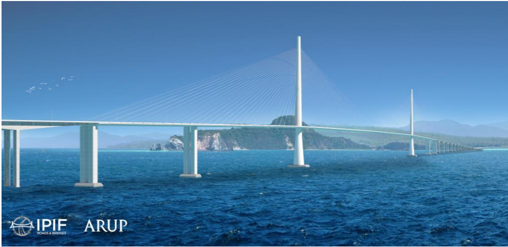
South Channel Bridge
