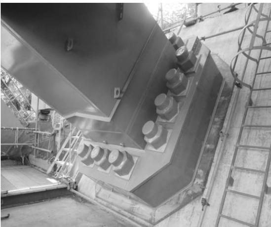
Figure 24. Arch base for improved durability.
