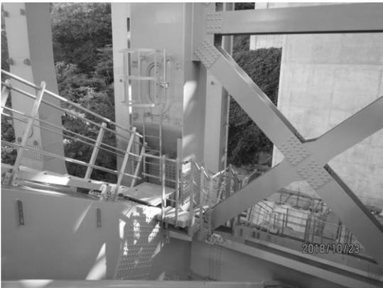
Figure 20. Inspection road of superstructure.
