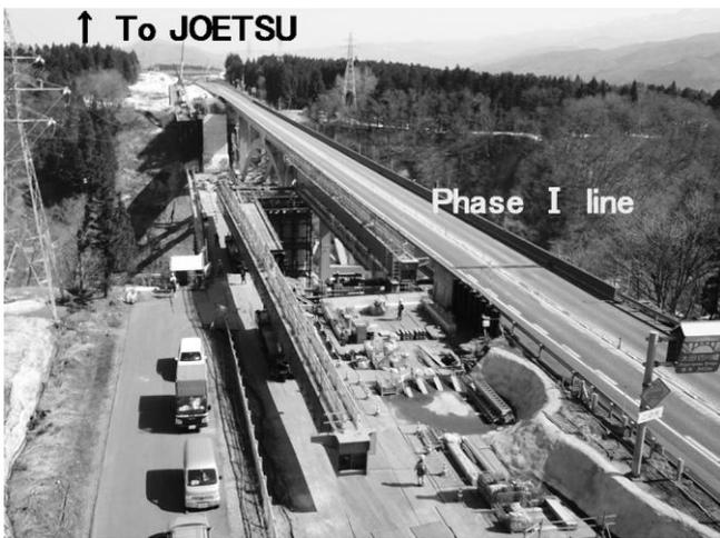
Figure 11. Transportation by multi-axle trolley.
