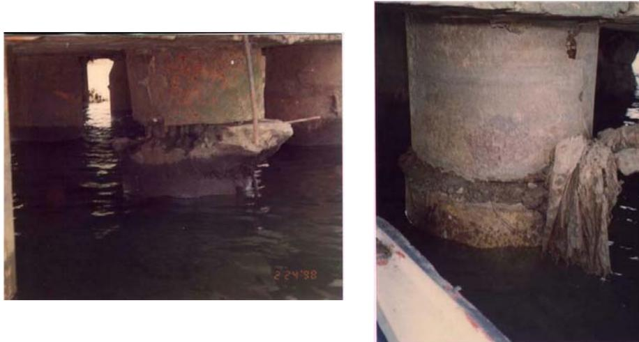
Fig. 3. Photograph shows defective concrete work in the piles for Dhaleshwari-I Bridge.
