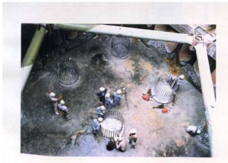
Fig. 2. Pile head treatment for construction pier foundation inside the cofferdam.
