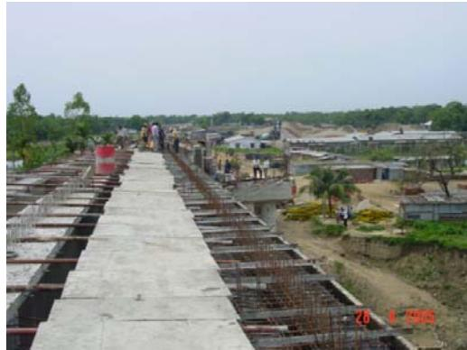
Photo 1. Under construction Sylhet Shah Paran Bridge showing precast deck forms
